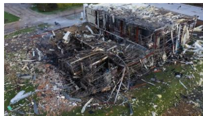
Mixing of Incompatible Materials: Evolved H_2 Explosion
