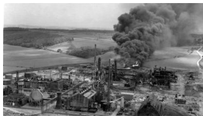
Pipework Failure: Cyclohexane VCE
