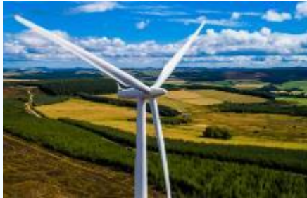
25.7MW onshore wind farm, expected to generate c.70GWh per annum from around 2027 at Bridgend
